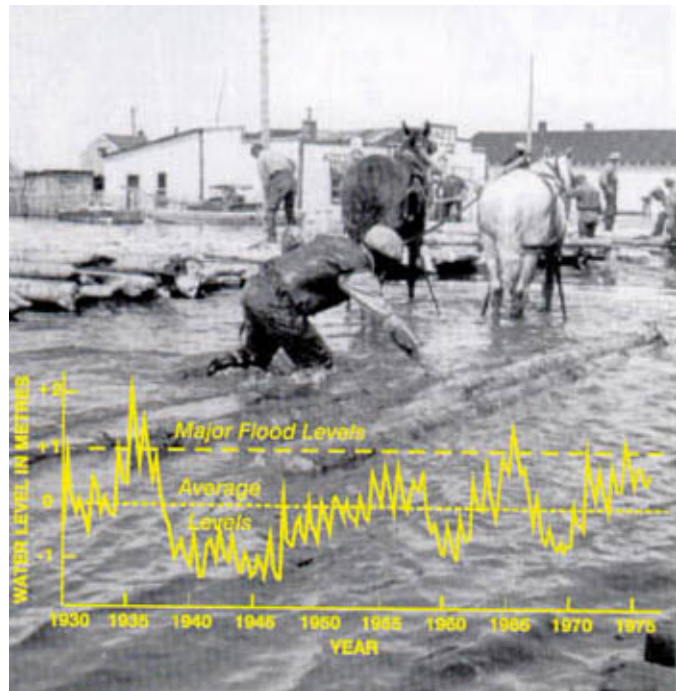
Figure 46: Constructing an elevated log road along the main street of Sawridge (a town adjacent to Lesser Slave Lake) during the historic flood of July, 1935). A 30-year plot of annual flood peaks is super-imposed on the scene (photo courtesy R.W.H. Eben-Ebenau: lake levels from Nemanishen and Cheng").
