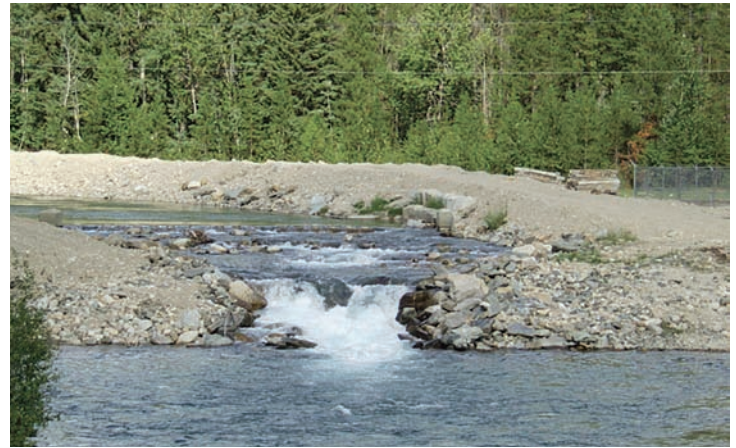
The rushing waters of Swift Creek will provide the community of Valemount with clean water with the help of their new water storage and filtration system.
