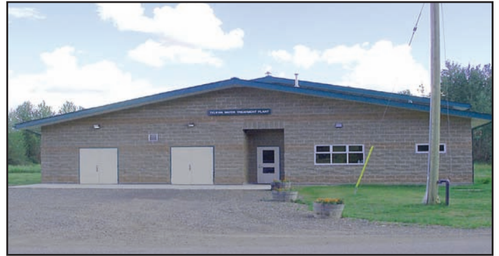
Telkwa's new water treatment plant, which includes new water filtration technology, delivers clean drinking water to over 500 households across the community.
