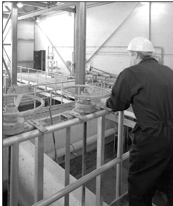
Inspection and management of our infrastructure
