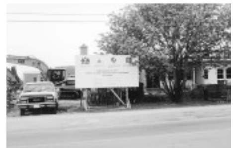
The London school-community centre under construction.
