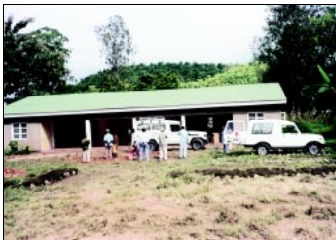
Lusanga dispensary after rehabilitation.
