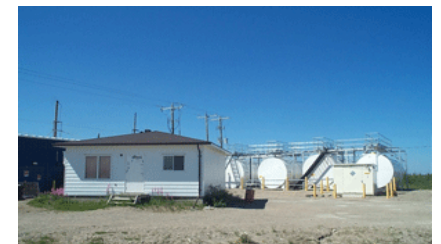
Habitation Hydro One - PN Fort Severn
