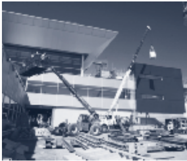
Construction work at Pierre Elliott Trudeau International Airport in Montréal
