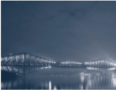
The Quebec Bridge at night.
