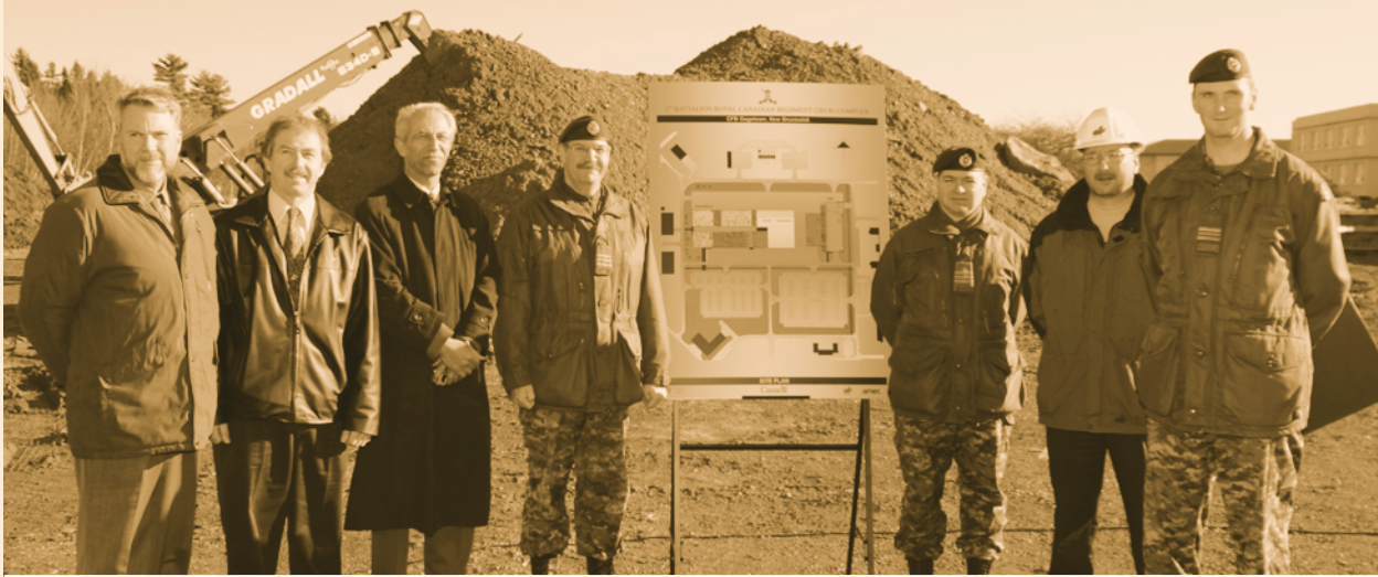
In November, 2003, DND announced the construction of the 2 nd Battalion Royal Canadian Regiment's (2 RCR) new Garrison Facility at CFB Gagetown. DCC is providing contract management services for this $11 million project. Pictured above from left to right: Robert Guthrie (Architect, AMEC), Darrell Stewart (Contract Coordinator, DCC), Sia Salehi (Project Manager, DCPEP 4-2), LCol Bruce Parks (CO Eng. Branch 3ASG), LCol R. Turcotte (DCPEP 4), Albert Madsen (Site Manager, DCC) and Maj. Peter Burgess (RA-DEV 0 3ASG).
