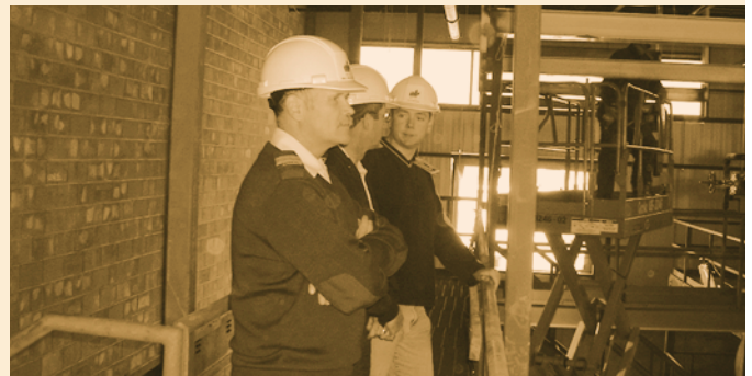
DCC Engineer, Trevor Rogers, escorts DND personnel through the Central Heating Plant 3 at CFB Greenwood.
