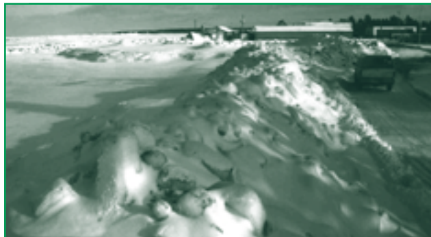
Ice thrown onto the shoreline by the January 21, 2000, storm surge destroyed a building and nearly closed a road in Robichaud, New Brunswick, on the southern shore of the Gulf of St. Lawrence. Photo: Donald Forbes
