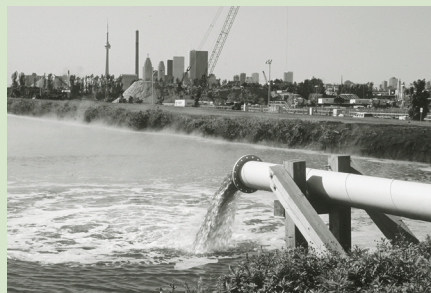
Sewage lagoon near Toronto
