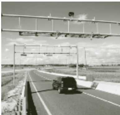
Toll collector devices for vehicles merging onto a toll roadway
