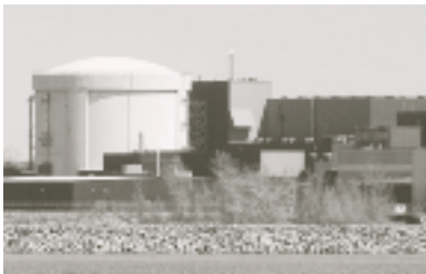
Gentilly-2 Nuclear Generating Station
