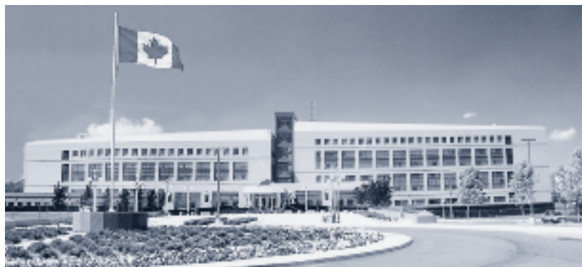
The Canadian Security Intelligence Service (CSIS) National Headquarters. CSIS, along with the other organizations mentioned in this chapter, contributes to Canada's security.
