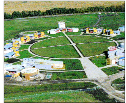
Cover photo The new minimum security Aboriginal facility at Hobbema, Alberta
