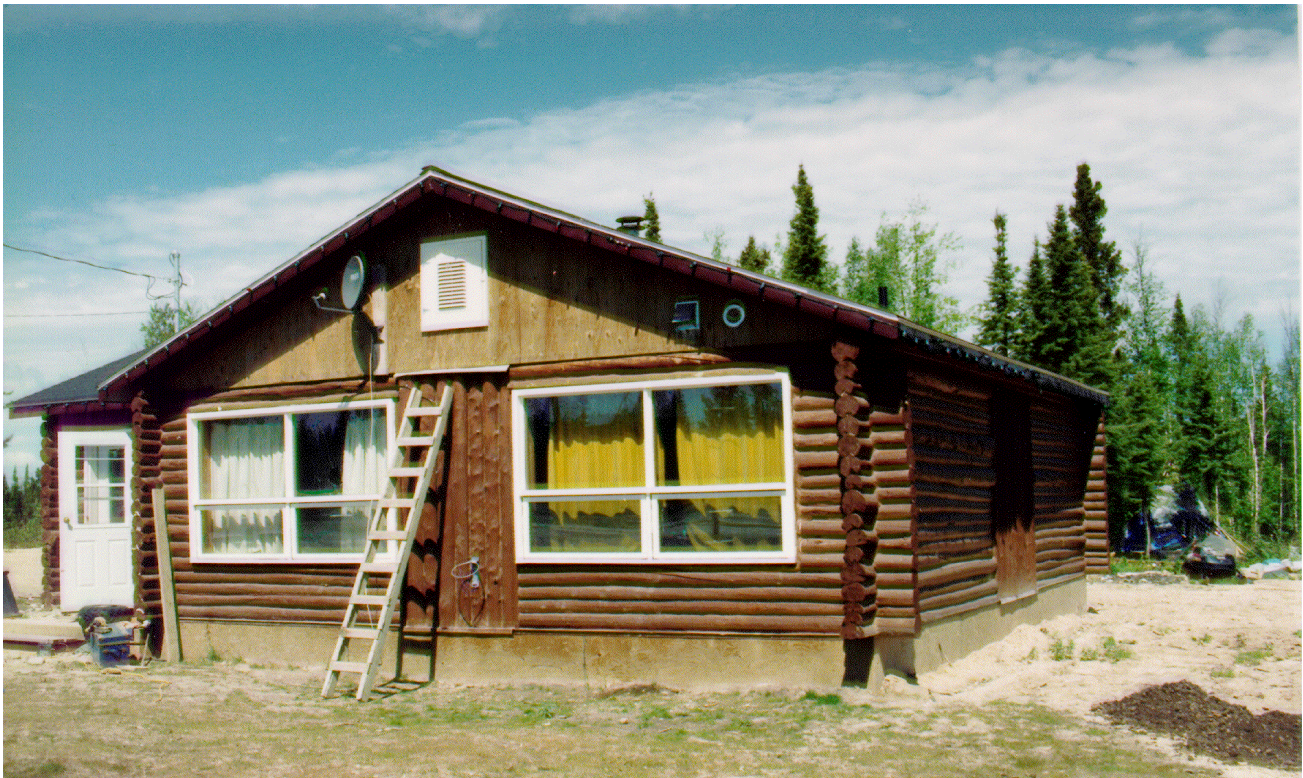
Figure 1: The four log houses built at Big Trout Lake used a combination of vertical and horizontal logs.
