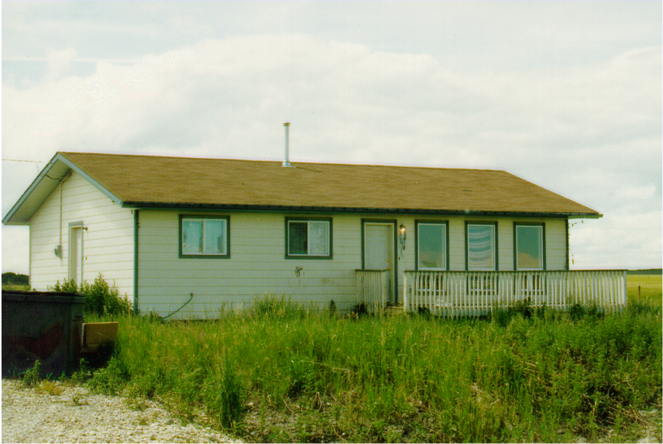
Figure 4: One of the five stud-framed houses built at Tsuu T'ina during the pilot project.
