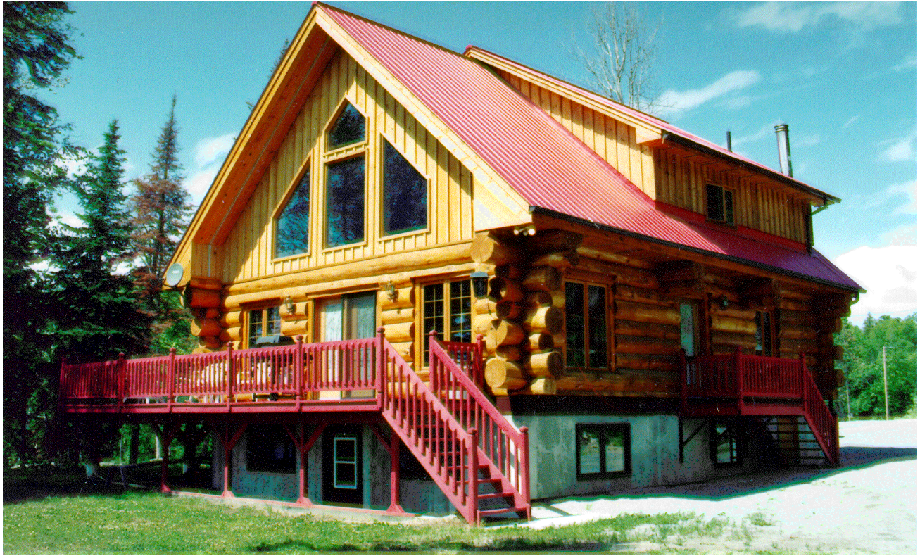
Figure 2: Five Scandinavian style log houses were built at Kitigan Zibi. The owners of each log house selected the overall design and layout of their log homes.
