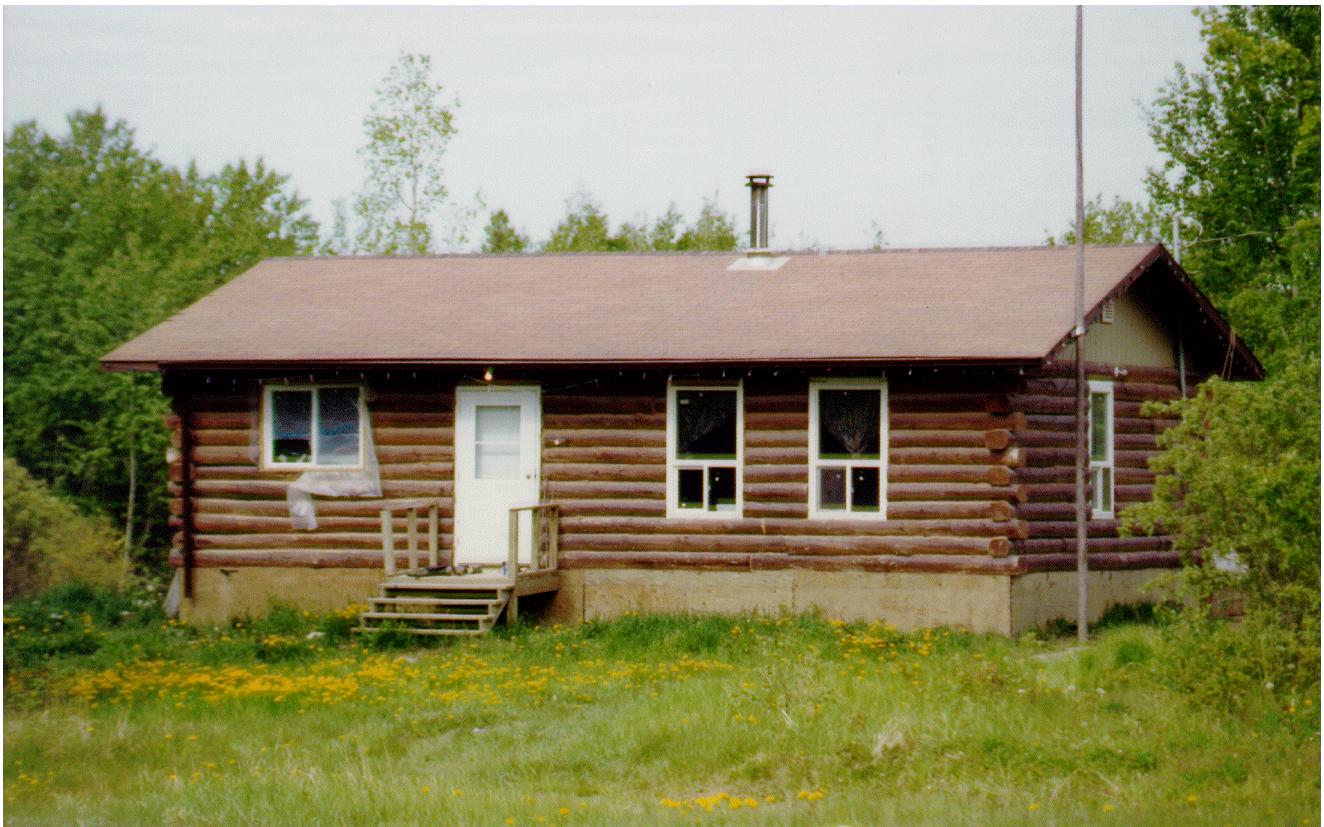
Figure 3: Five houses using a milled-log process were built at Sandy Lake. Only the exterior of the house resembles logs.
