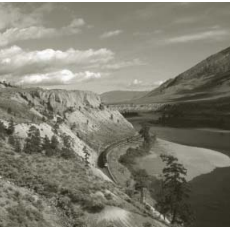
Aerial view of a westbound train near Kamloops, British Columbia 1975
