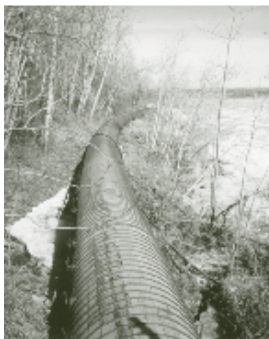
Outfall pipe leading to the Winnipeg River at the Pine Falls Pulp and Paper Mill, Manitoba.
