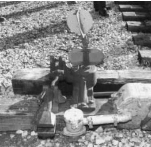
West crossover switch, Mile 46.72, lined and locked in 1'the reverse position.
