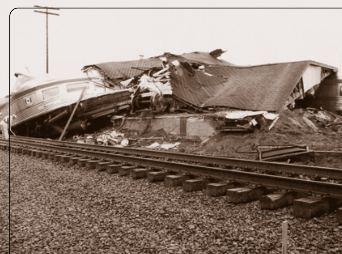
Damage to diner car and farm supply building. Note foundation wall and roof of building in centre of photograph.
