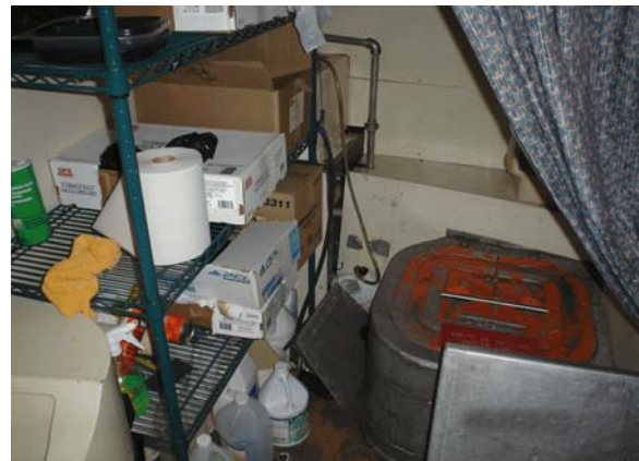
Photo 4. Unsecured stores near the starboard engine room escape hatch
