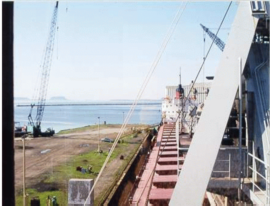
Photo 2. Starboard side of bridge looking aft
