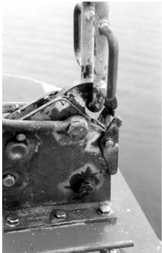
Photograph 9. View of hook, suspension ring, and retaining latch
