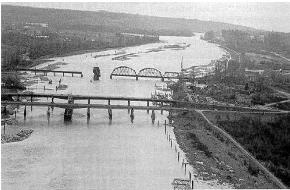
Photo 2. River Bridges looking downstream (1986)
