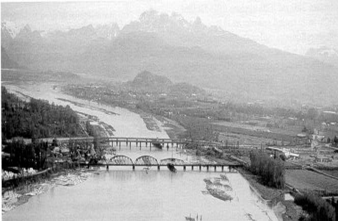
Photo 1. River Bridges looking upstream (1999)
