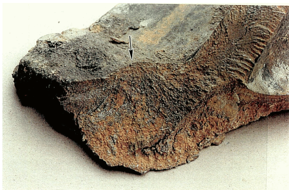
Photo 4. Close-up of fracture initiation location in thermite weld
