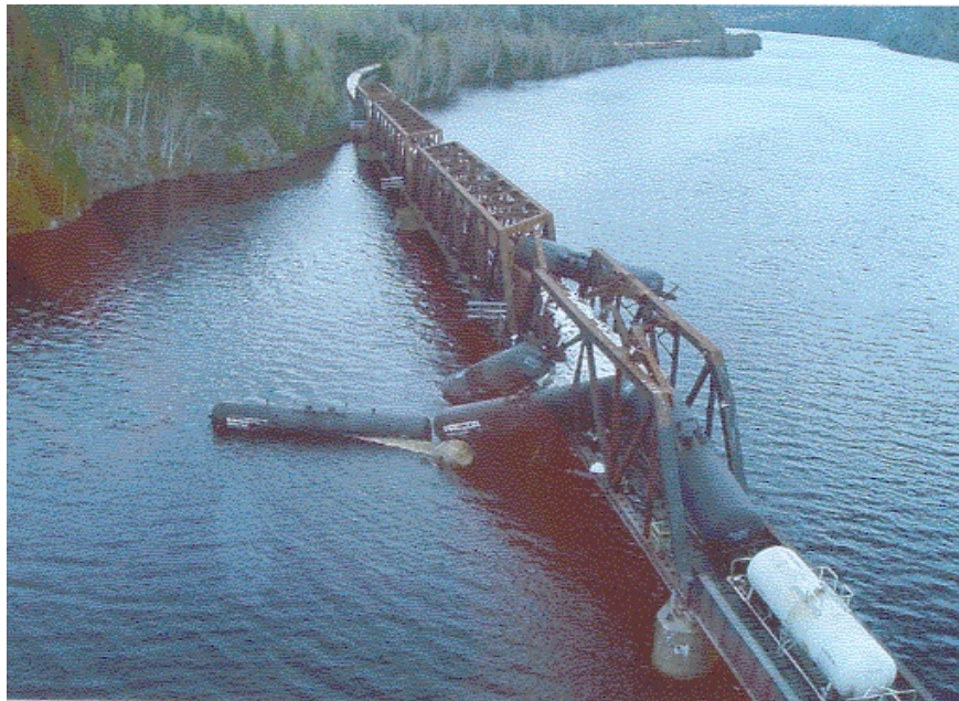
Figure 2. View of derailment on the bridge (72nd to 80th cars)
