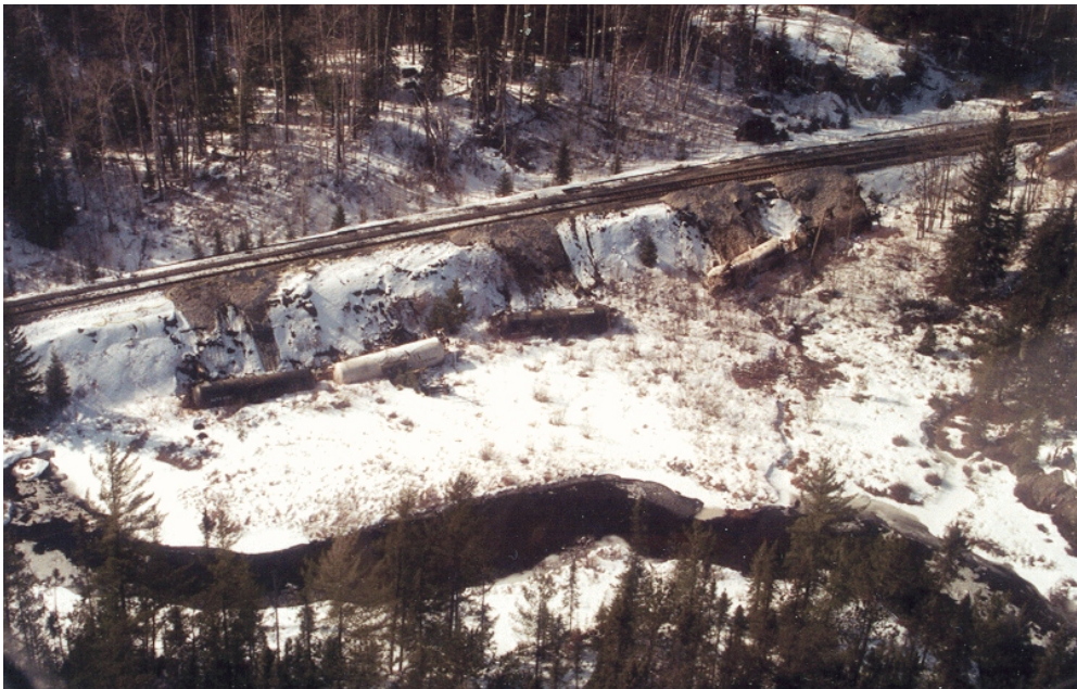
Figure 2 - South end of derailment site
