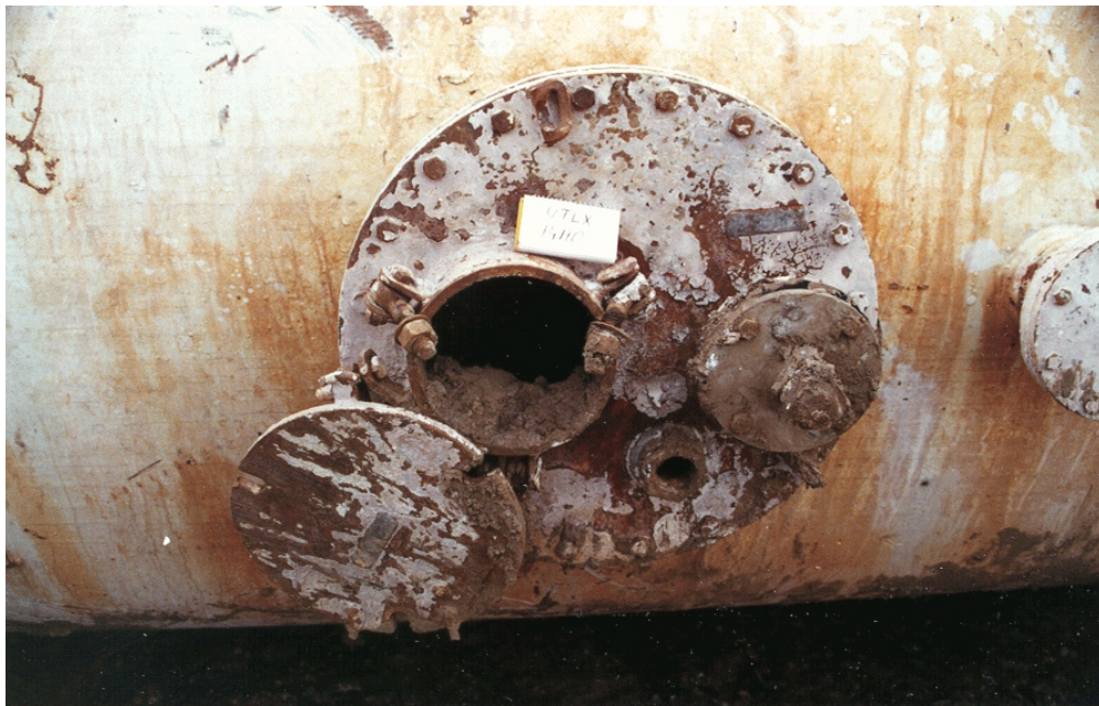
Figure 4 - Top fittings sheared off during the derailment
