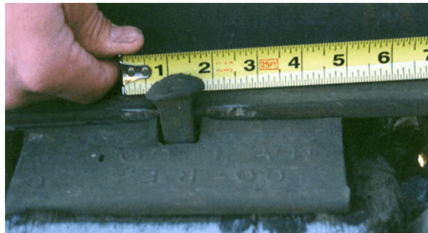
Photo 3. Indicator of track movement
