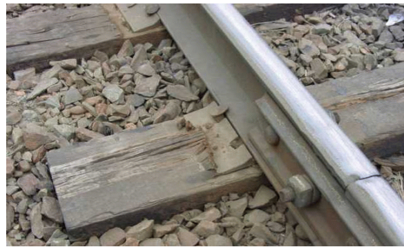
Photos 1 and 2. Track conditions near the initial point of derailment, including plate-cut ties and spikes.
