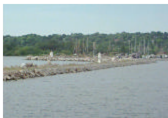
Bay Port's Environmentally Friendly Break Wall
