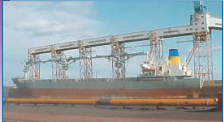
Bulk Carriers calling in Canada, which meet criteria for the Bulk Carrier Inspection Programme, may be given a special inspection including the vessel's structure
