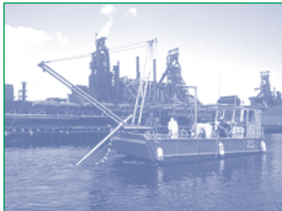
LIST being used in a pilot-scale remediation project in Hamilton Harbour.
