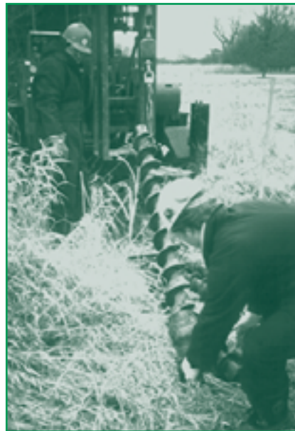
Installing a multi-level groundwater sampling well in Point Pelee marsh.
