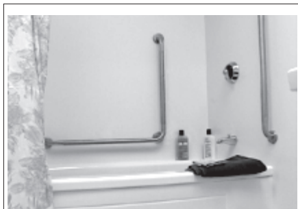
Seniors should have grab bars in all bathrooms, as well as non-slip mats in and beside the tub. A bath seat or bench is often very helpful.
