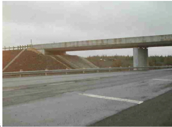
New Arnold's Cove Overpass
