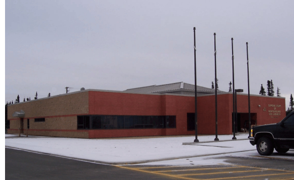
New Courthouse in Happy Valley-Goose Bay
