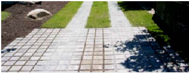
Permeable paver lane entrance
