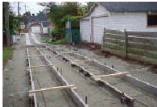
Concrete driving strips being built
