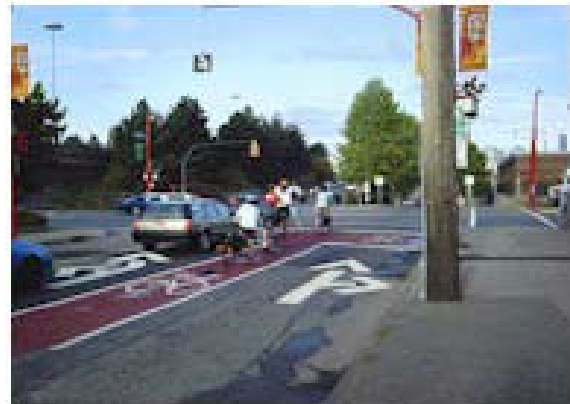
New "Bike Box" pavement markings with a cyclist advance red light
