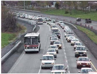
Freeway shoulder bus lane in operation
