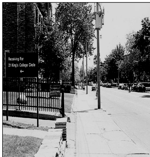
A section of St. George circa 1994. The street had fallen into disrepair and was in need of rehabilitation.
