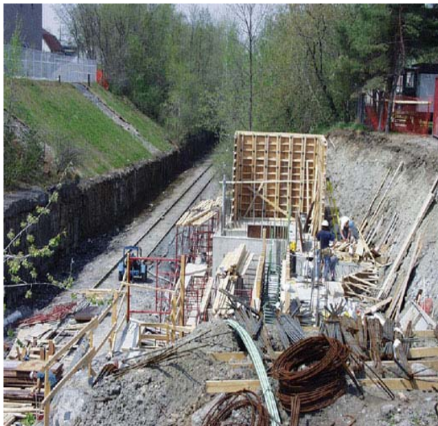
The Carling Avenue station under construction.
