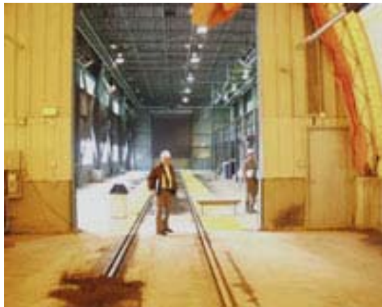
A prefabricated structure at the Walkley Road maintenance facility houses the trains
