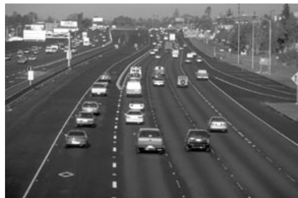
High-occupancy toll lane (with diamond markings, left) on I-15 in San Diego, CA (Source: U.S. Federal Highway Administration)
