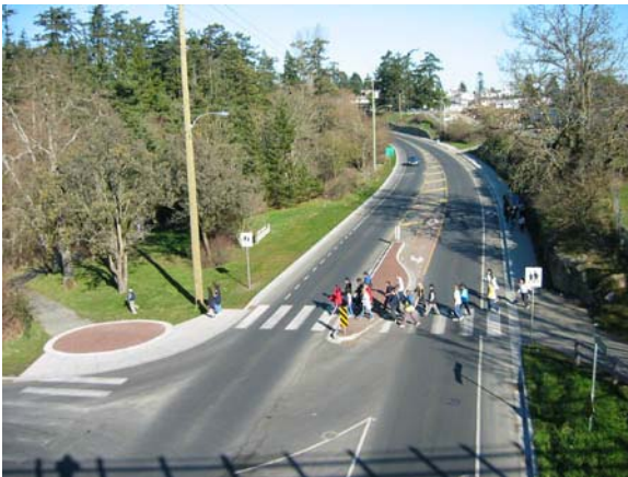
Improved sidewalks and cycling lanes with dedicated bike turning bays near the University of Victoria.
