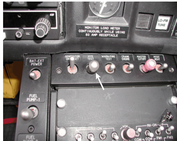
Photo 3. Hydraulic HYD TEST switch
