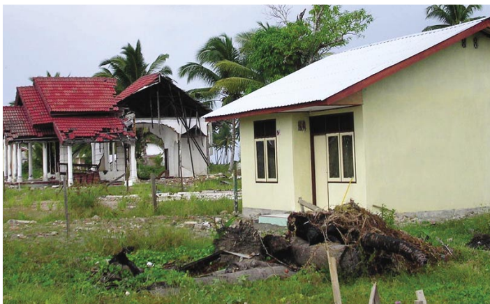
One of many houses that have been built
