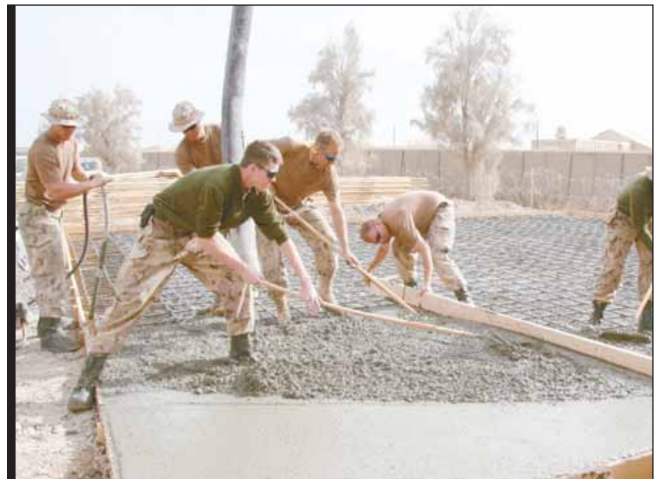
Troops from 191 AEF (Comox), 192 AEF (Abbotsford), and PNCT (Esquimalt) pour concrete for an extension to the TOC building in Kandahar, Afghanistan.
