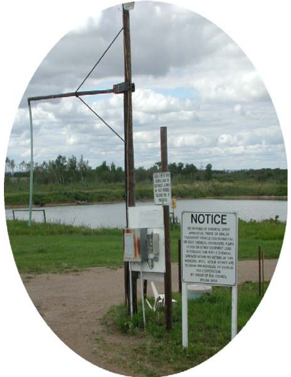
Tank-loading facilities provide people with access to community projects supplying drinking water or raw water. Responsibilities differ for both kinds of water.
