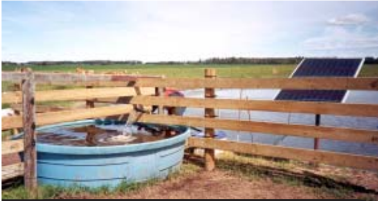
Excess power produced by solar panels can be used to aerate a dugout or power an electric fence
