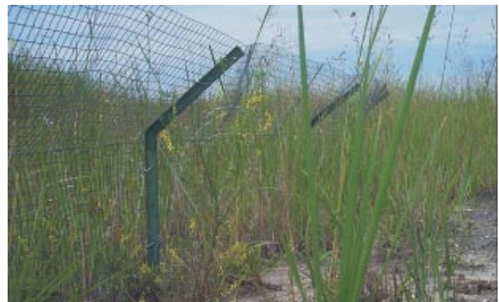
A wire mesh fence has been used to keep muskrats out of wetlands.
