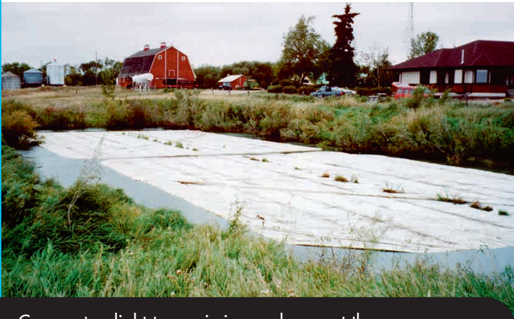
Covers stop light transmission and prevent the growth of algae. They also reduce evaporation
