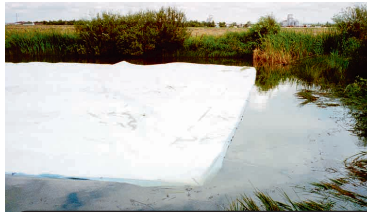
These covers float with submerged skirts, and are anchored to the shore at each corner
