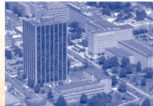
Natural Resources Canada's Booth Street Complex, Ottawa.
