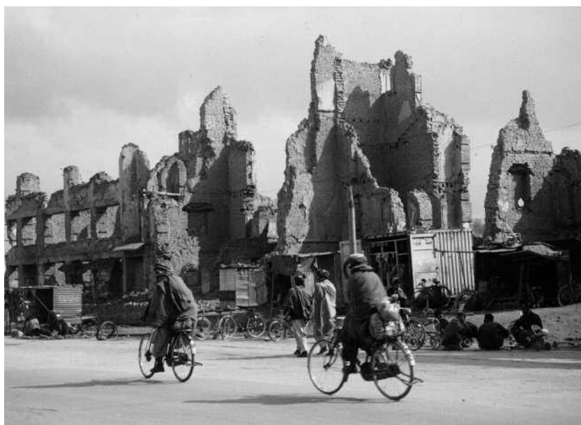
Damaged housing in Kabul, Afghanistan. © R. Warah/UN-HABITAT
